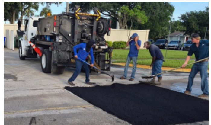
Asphalt repair operation with crew placing and leveling hot-mix asphalt.
