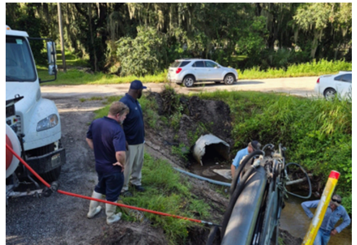
Culvert and ditch maintenance/repair using vacuum and excavation equipment to restore drainage function.
