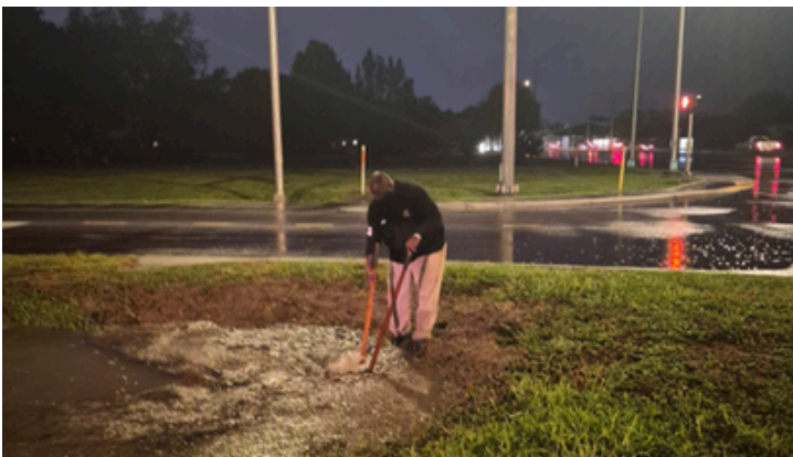
After-hours drainage response at a signalized intersection during wet weather conditions.
