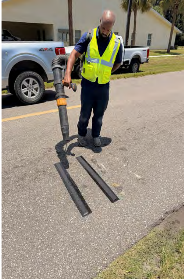
Adding Rumble Strips on NW 9 th street
