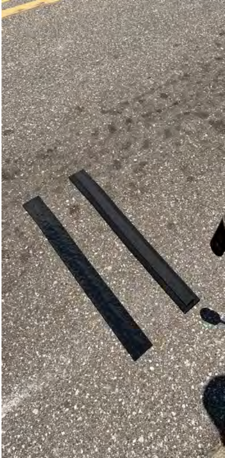
Adding Rumble Strips on NW 9 th street
