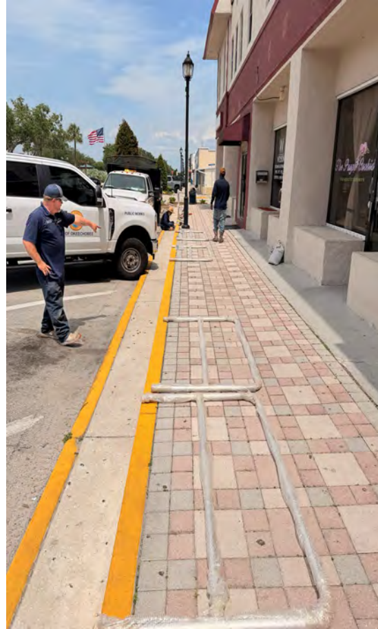
Installing Handicap Rails on Park Street
